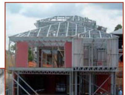
Steel frame construction
