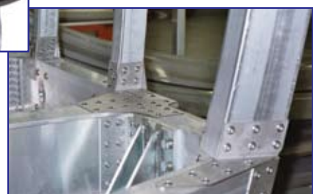
Train Wagon Assembly / Repairs
